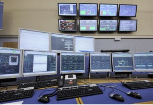
Total SCADA: The universal process control and visualisation system, PVSS, in the Central Control Centre at CERN ensures trouble-free control and monitoring of the particle accelerator's entire technical infrastructure in a homogeneous user interface
